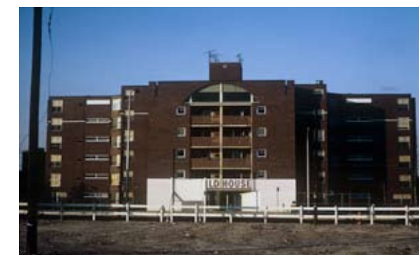
Guild House, Venturi and Rauch
