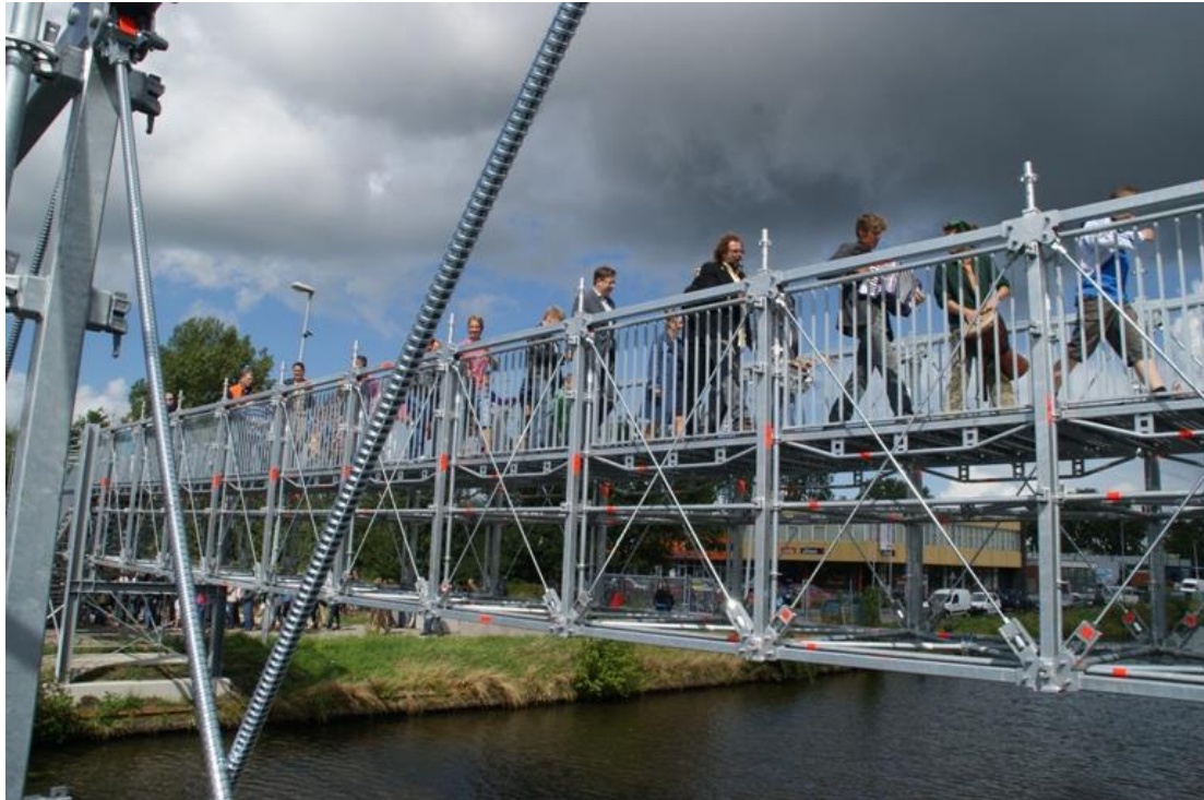
Temporary bridge on the Hoendiep, first prize Europan 12, Groningen, Elizabeth Keller en Remco Roolvink
