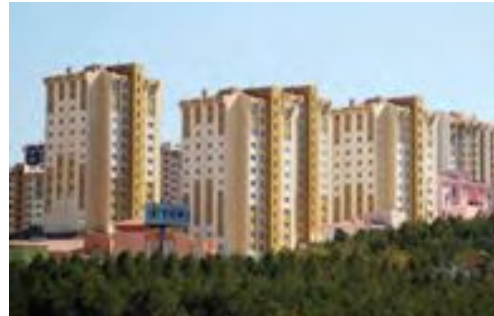
↓ An example of a TOKİ housing development
