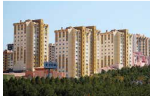
↓ An example of a TOKİ housing development
