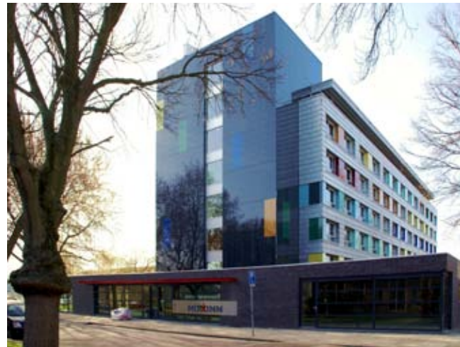
Mixx Inn, The Hague | Photograph A3 architecten
