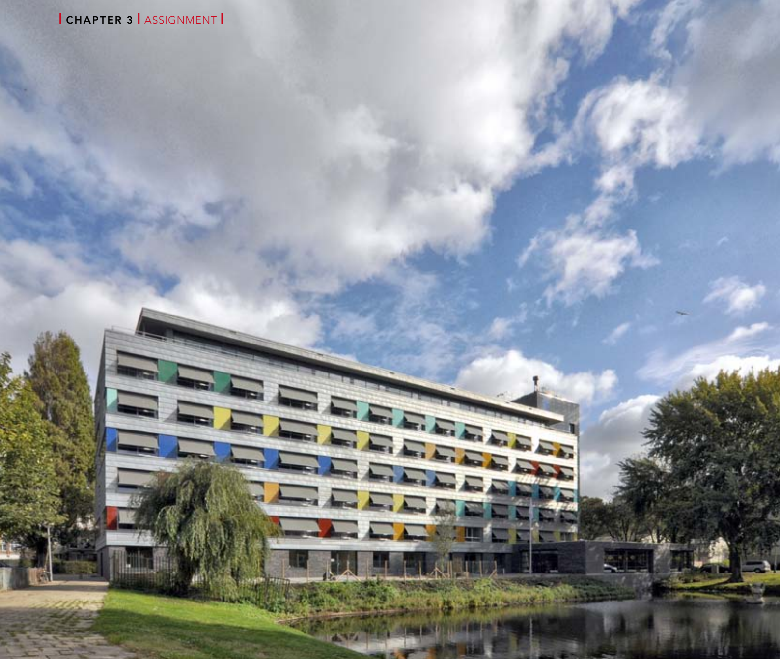
Mixx Inn, former nursing home in The Hague, now shortstay facilities | Photograph A3 Architecten
