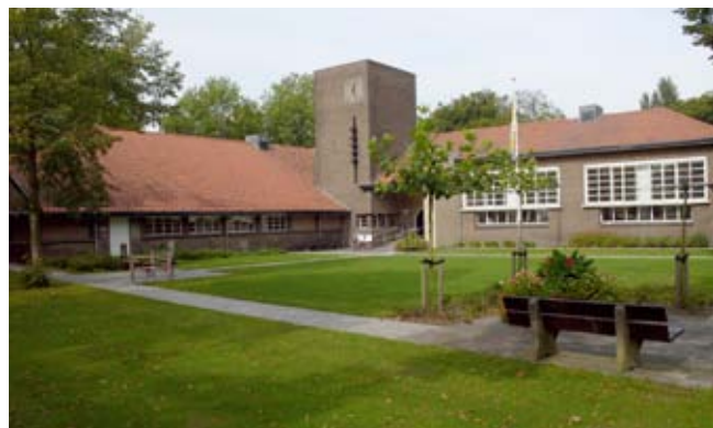
De Plataan, Amersfoort, former school | Photograph Jos Sikking
