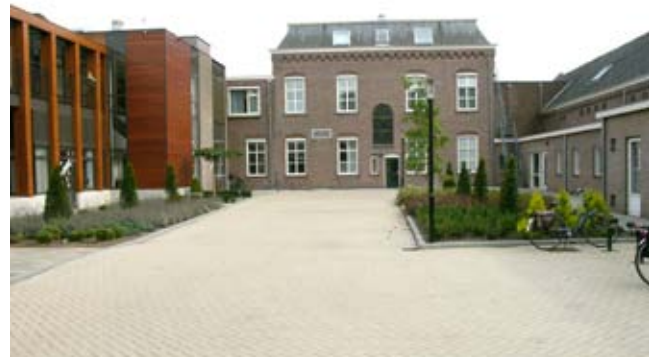
Haarenstaete, former monastery, now a residential care centre, Mariaheide | Photograph Jos Sikking
